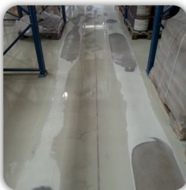
Track after grinding the high points
