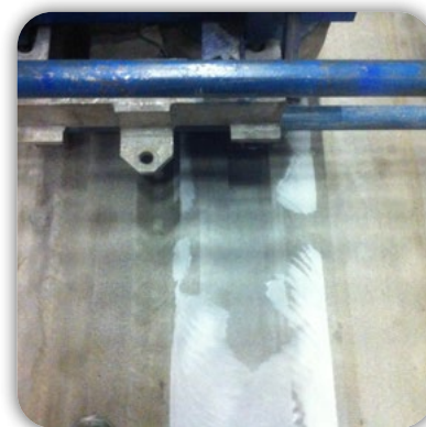
Detail picture high point grinding
