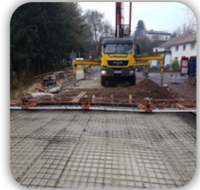
Electric screed with W profiling - 3 inclination changes
