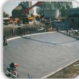
Round clarifier with 15 m span
